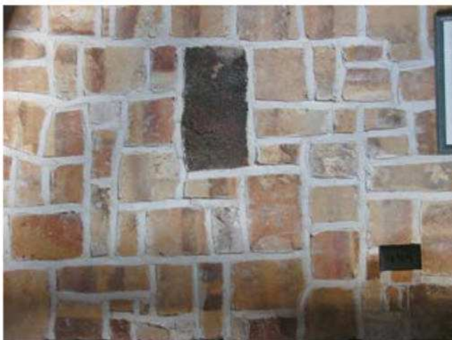
Above: Two interior walls made with salvaged bricks. The top ones are from the Whangarei Window Glass works, some with glass embedded.
